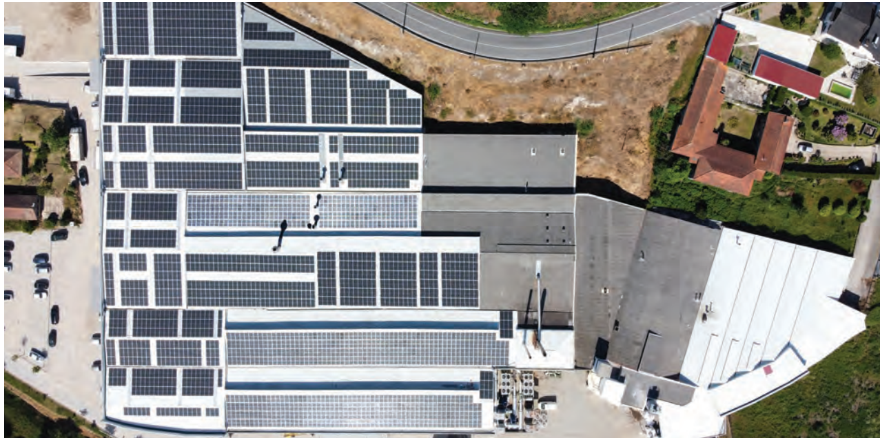
Using the sun for sustainability. Reduction of 265 Ton CO 2 per year with 420 kW of photovoltaic panels for self-consumption.
